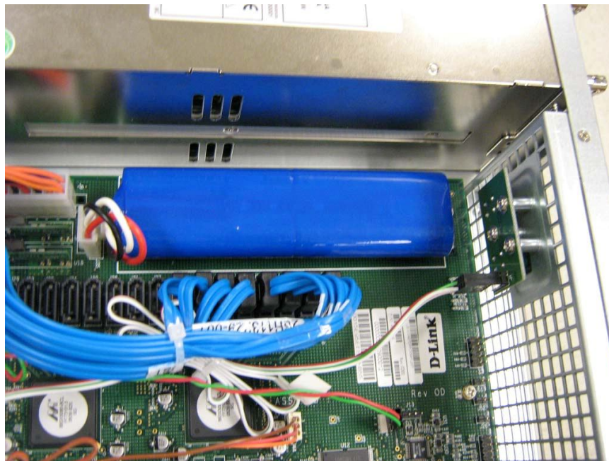
Figure A-5 The Installed Battery
